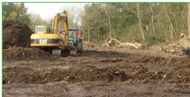
Deforestation and removal of debris and top soil to restore humid dune slack
