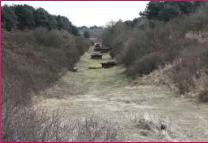
Older drainage canals are now used for the collection of water from the infiltration system.
